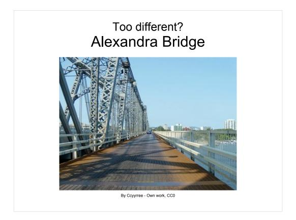
...which has an additional road lane tacked onto one side and a walkway tacked on to the other.
